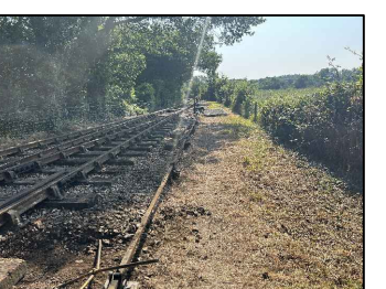
VIEW 4: UPLINE FROM CHAINAGE 200
