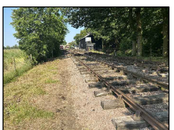
VIEW 3: DOWNLINE FROM CHAINAGE 180
