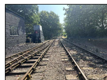
VIEW 2: UPLINE FROM CHAINAGE 80
