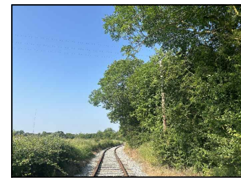
VIEW 10: POWER LINE FROM 700
